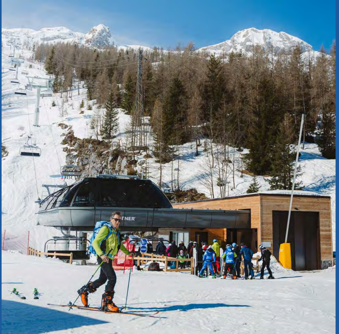
Colere. View of the chairlift system at the level of the intermediate station.
